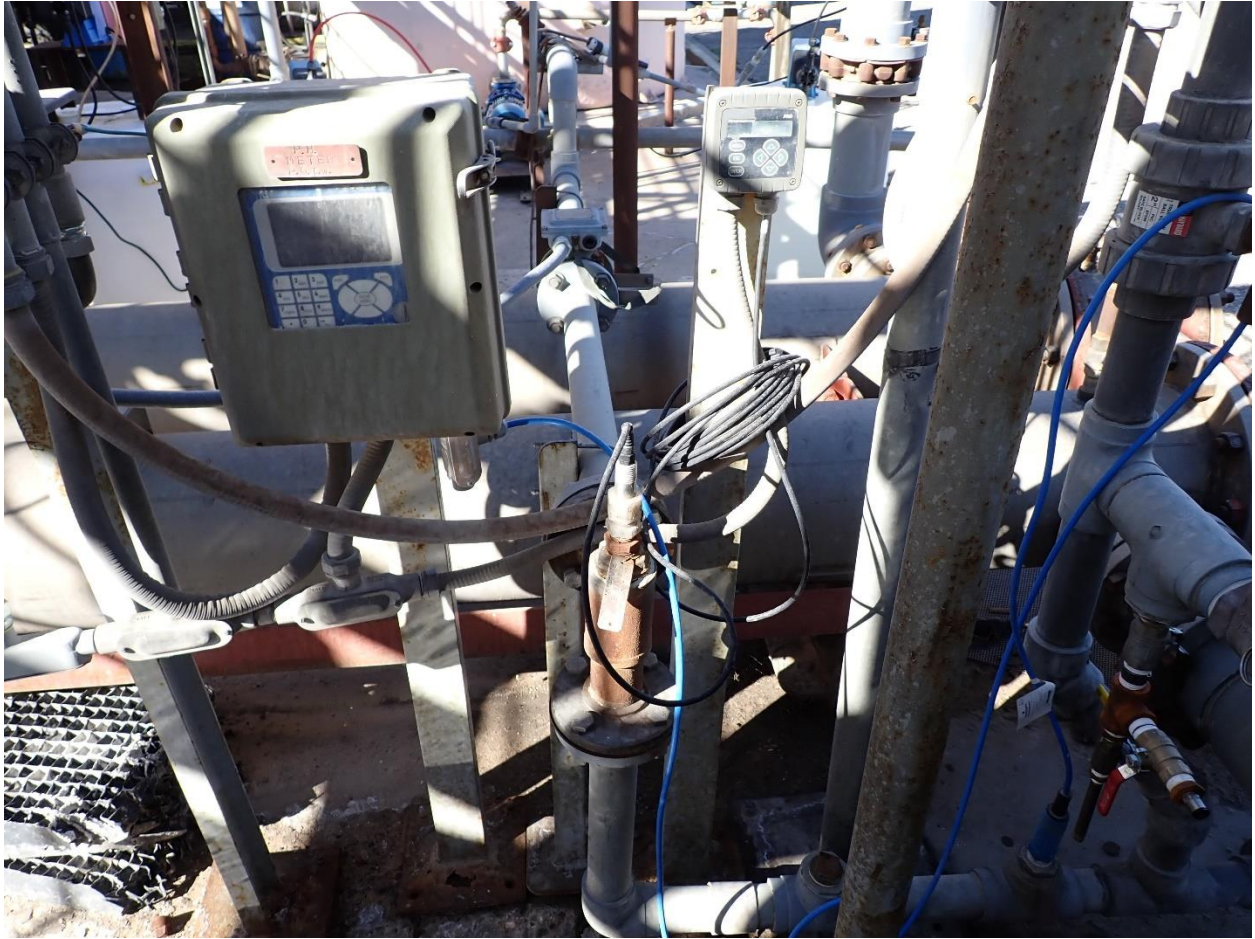
Photo 8: Sampling point for pH and TDS
