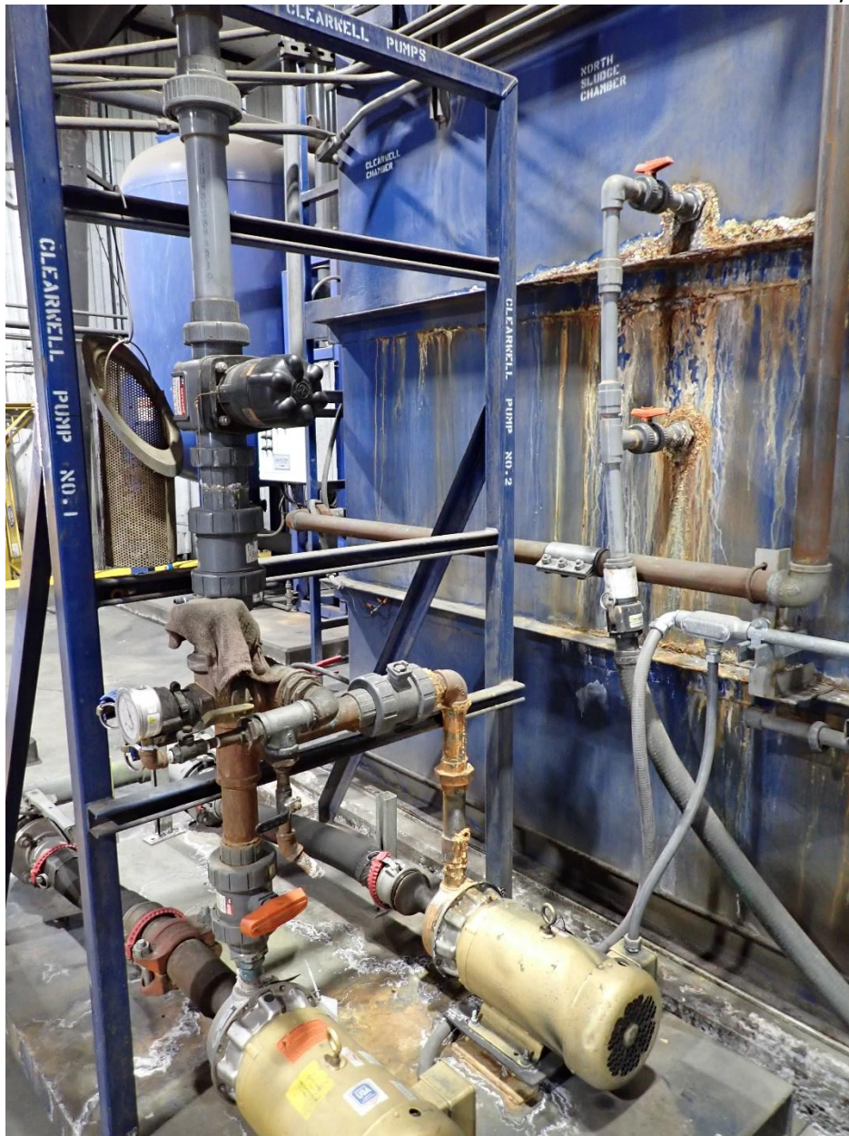
Photo 4: Clearwell chamber. Floor drains lead to the wastewater treatment system.
